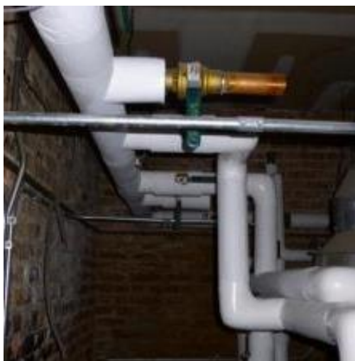
Insulate 100% of hot water pipe
