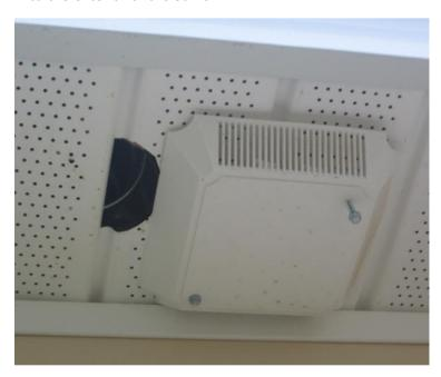
The vent is extended to the soffit but not extended and permanently affixed through the soffit.
