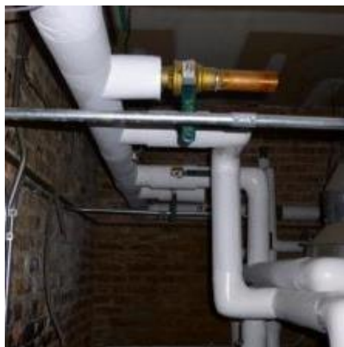
Insulate 100% of hot water pipe
