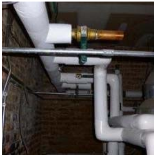
Insulate 100% of hot water pipe
