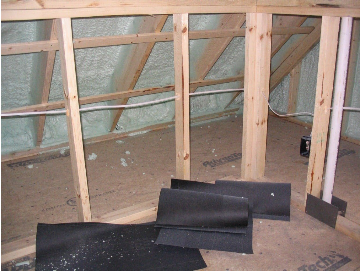
Photo Image of spray applied foam insulation along roof decking.
