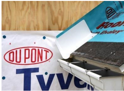
Step 2: Install shingle starter strip, then kick-out flashing. Secure to roof deck but not to sidewall
