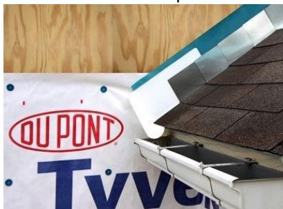
Step 4: Install flashing, counter flashing and shingles
