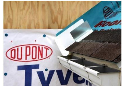
Step 3: Install first shingle and flashing over upper edge of diverter
