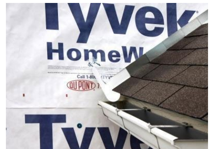
Step 6: Install next layer of housewrap to fit over top of diverter. Maintain at least a 2" exposure of step flashing.
