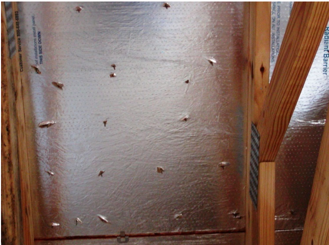
Radiant barrier material integrated with the roof decking.
