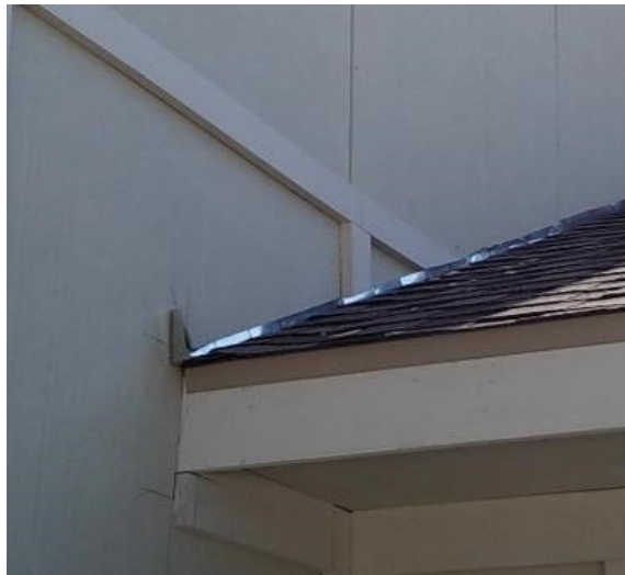
Flashing installed properly between roof and exterior wall.
