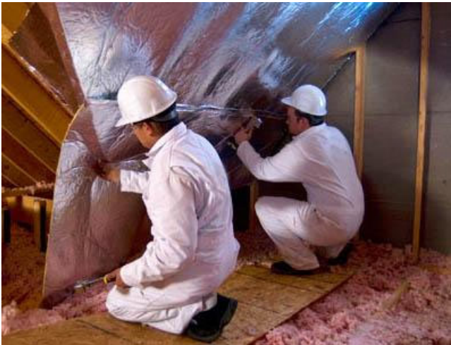
Radiant material can be retroactively installed to the underside of the roof truss.
