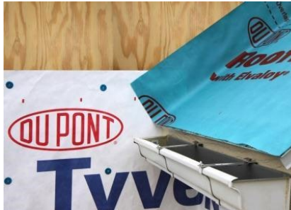
Step 1: Install roof underlayment (such as felt paper) over roof deck and up sidewall over housewrap
