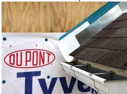
Step 4: Install flashing, counter flashing and shingles
